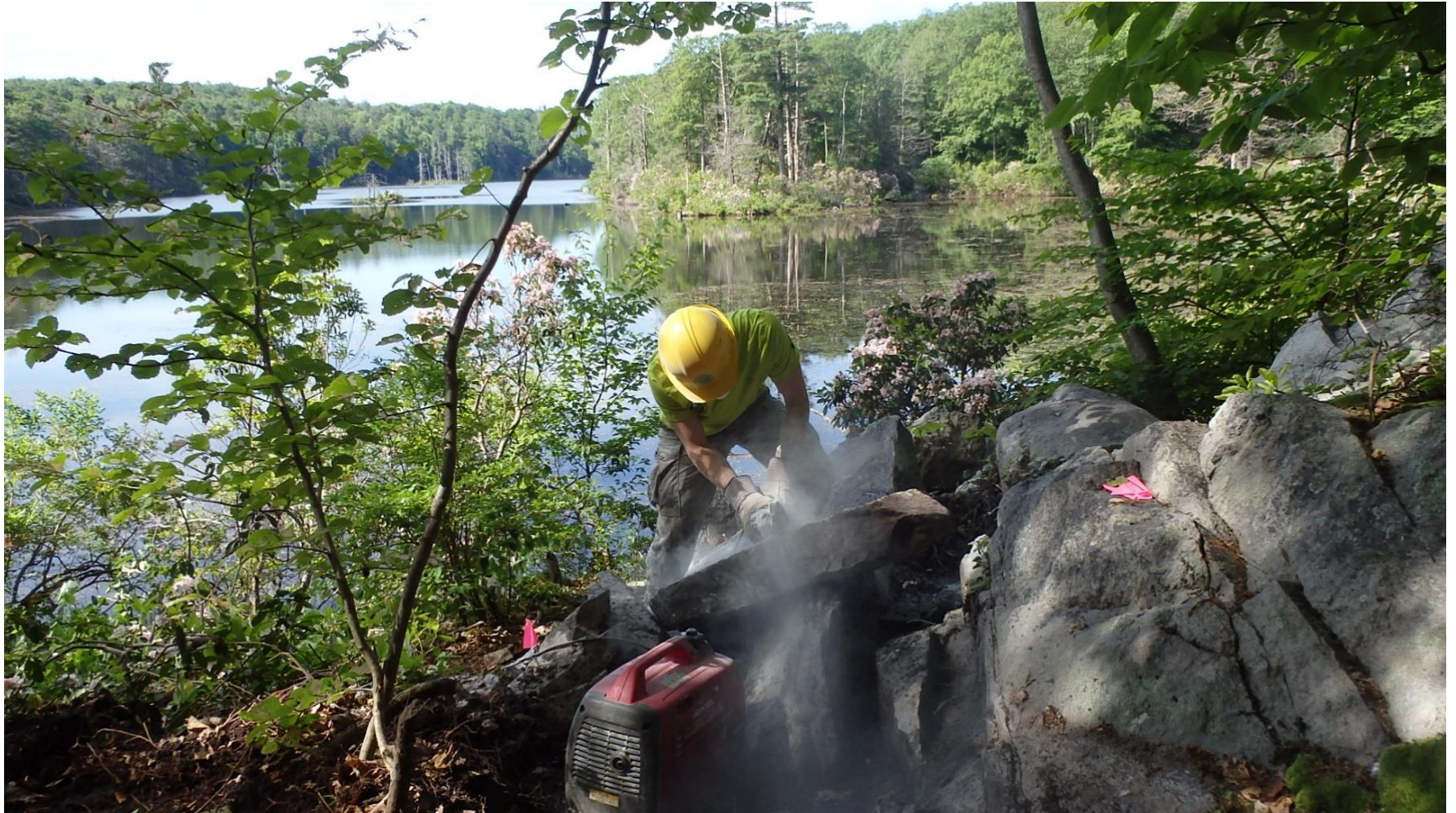
Cutting stone for steps
