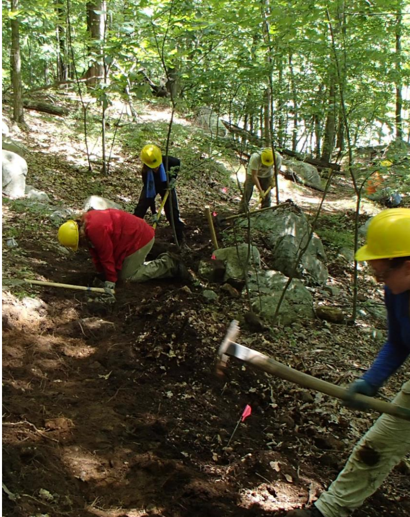
Volunteers cut sidehill.
