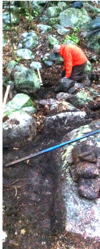
Tread elevated, paved and filled.
