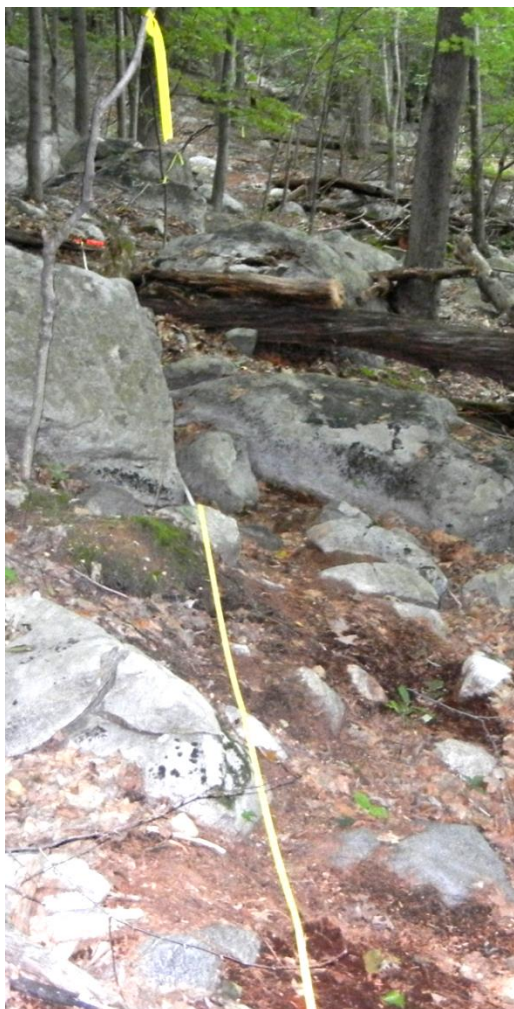
Retained, filled and defined tread.
