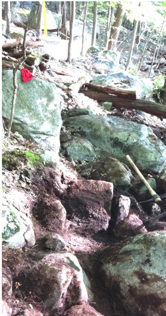
Retained, filled and defined tread.
