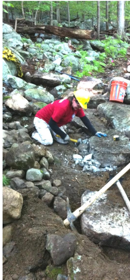
Area of intermittent flow paved.
