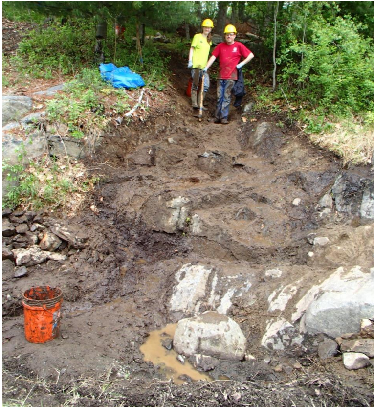
Bedrock exposed, drilled
